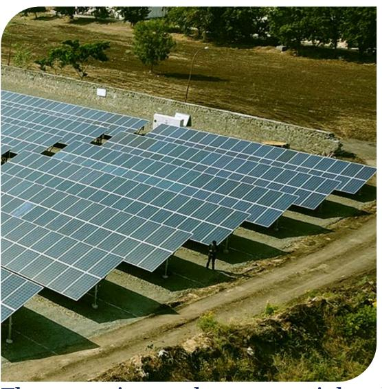
By installing solar panels directly on the ground rather than on rooftops, these projects maximize sunlight exposure and electricity generation. Ground-mounted solar arrays are especially well-suited for large-scale installations, such as solar farms, where vast expanses of land are available.
